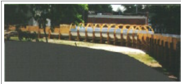
Figure 6. View of 220 degree cylindrical 90 degree Aeroduct curve sections to allow "banking" of the Aeromobile 17 at speed.
