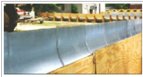
Figure 3. View across the Aeroduct ROW and the North straightway.
